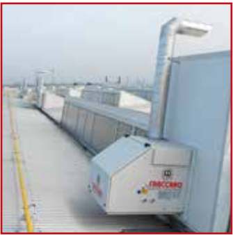
Installation en shed Sheddakmontage
